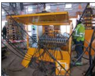
▼ Synchronous Stage Lifting: 48 double-acting jacks (25 and 50 ton) are networked in to a 16 points synchronous system to lift this 50 metres long, 1000 ton building up to a height of 2,5 metres to construct a new floor level.
