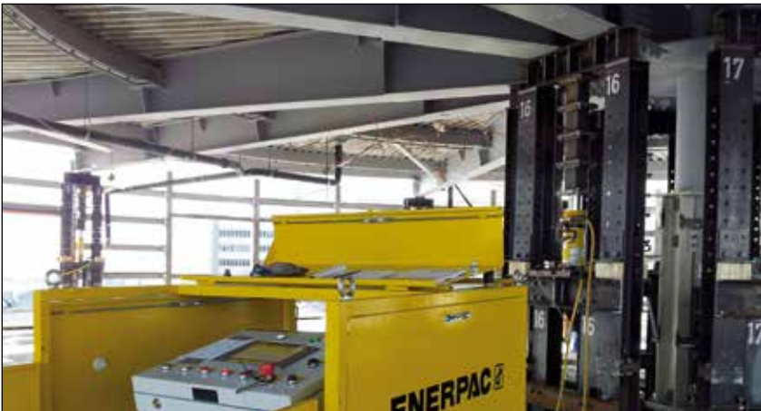
▼ Multipoint EVO-synchronous lifting system for roof support during construction.
