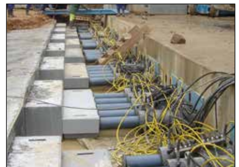
▲ Box jacking: Multi-point synchronous system to push hydraulically the tunnel segments under the railway.
