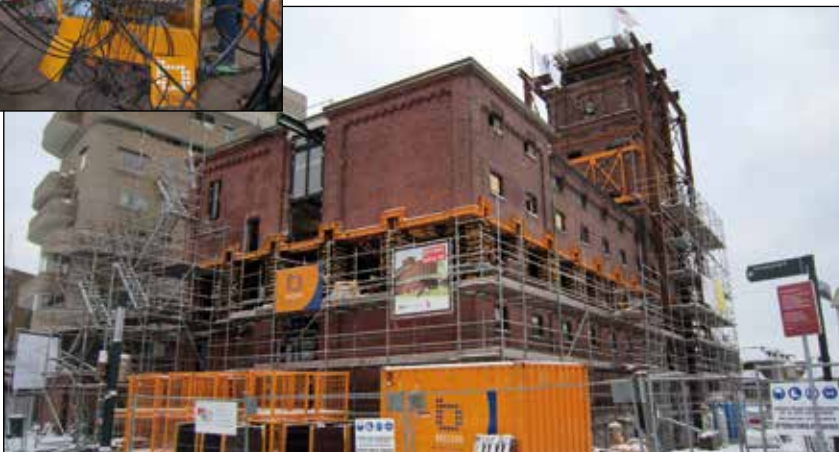
▼ Synchronous Stage Lifting: 48 double-acting jacks (25 and 50 ton) are networked in to a 16 points synchronous system to lift this 50 metres long, 1000 ton building up to a height of 2,5 metres to construct a new floor level.
